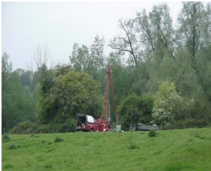
Borehole Drilling at Twyford Moors
